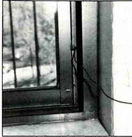
Fig. 2. Connection to metal window.
